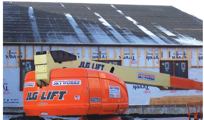
This exterior photo shows frost and snow still on the roof above the P2000 because heat did not escape and melt the frost. The heat loss through the fiber-glass area melted the frost on the rest of the roof.
