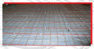
Insul-Tarp; as shown here, has been rolled out and installed with radiant tubing clipped to wire mesh.
