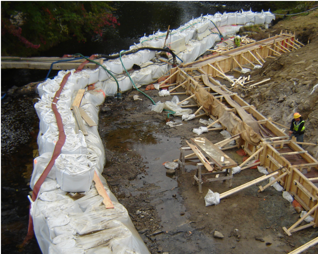
IVI Cubic Yard Bags are an effective solution when used as coffer dams during shoreline construction projects.
